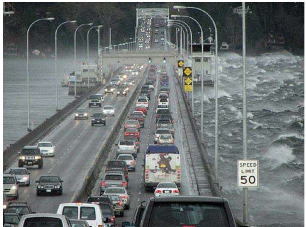
Figure 16.3.1 Floating Bridge, SR 520 Evergreen Point Bridge, Seattle, WA During Stormy Weather
