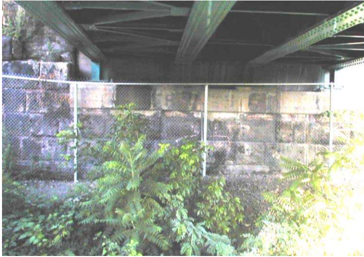
Photo No.5 North Abutment (far) - Elevation
