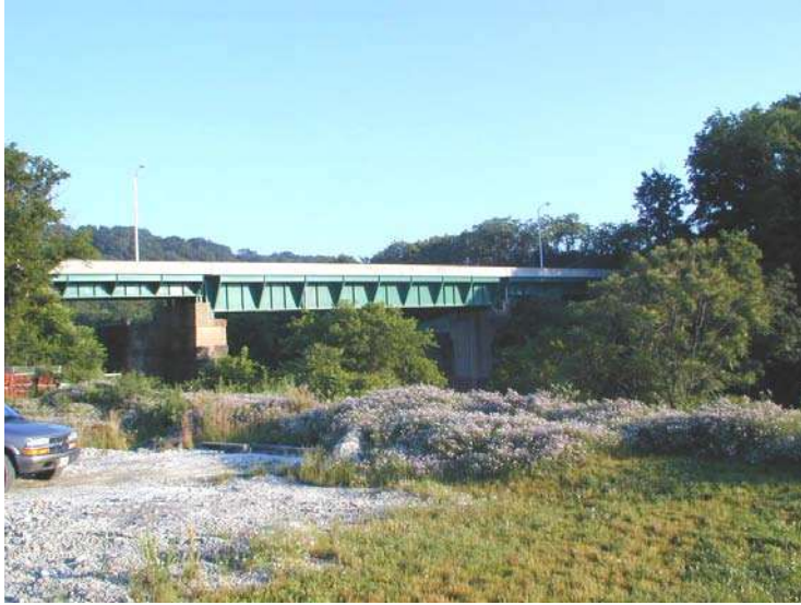
Photo No. 1 General Elevation (Upstream)
