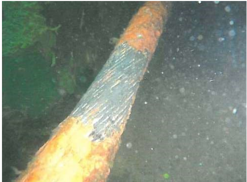
Figure 16.3.19 Typical View of Heavy Corrosion within Pontoon Port
