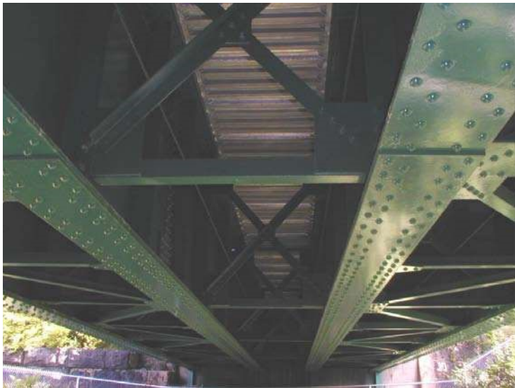
Photo No. 10 General Underside View – Span 3
