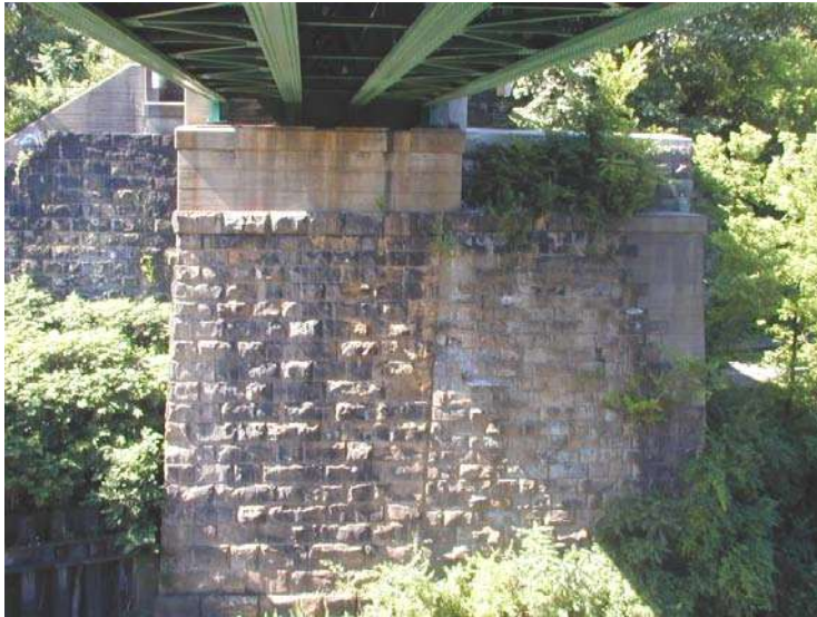
Photo No.6 Pier 1 - North Face (Looking South)
