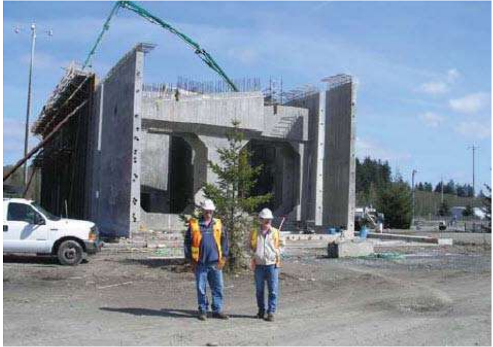
Figure 16.3.5 Concrete Pontoons Under Construction
