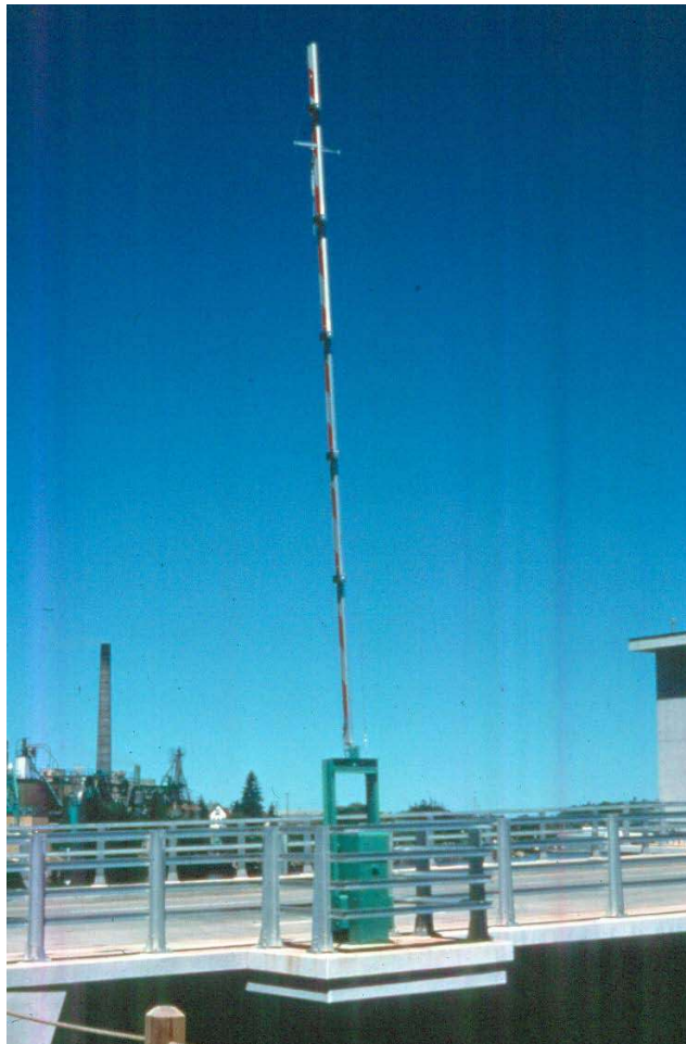
Figure 16.2.54 Traffic Control Gate
