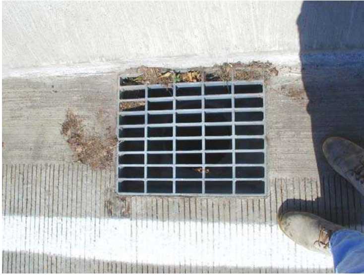
Photo No. 15 Typical PennDOT Type 1 Scupper
