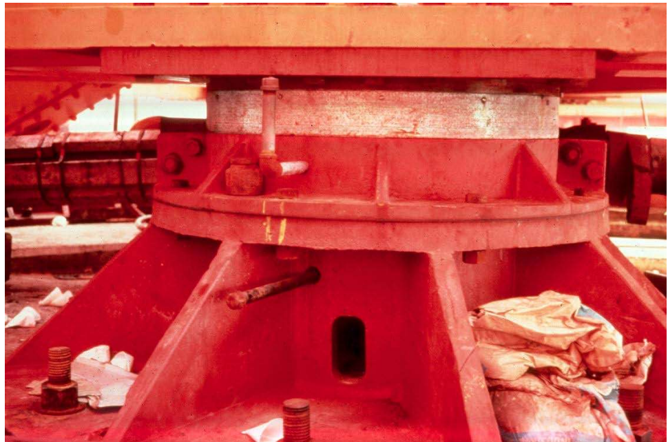
Figure 16.2.36 Center Pivot Bearing
