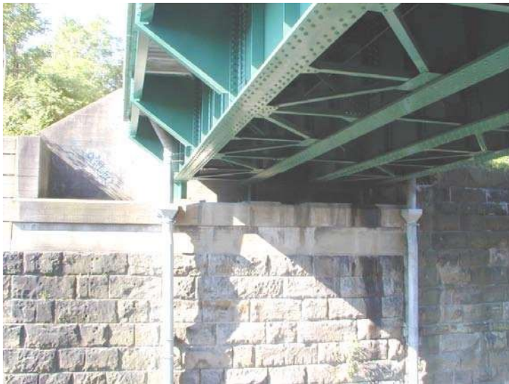
Photo No.4 South Abutment (near) - Elevation
