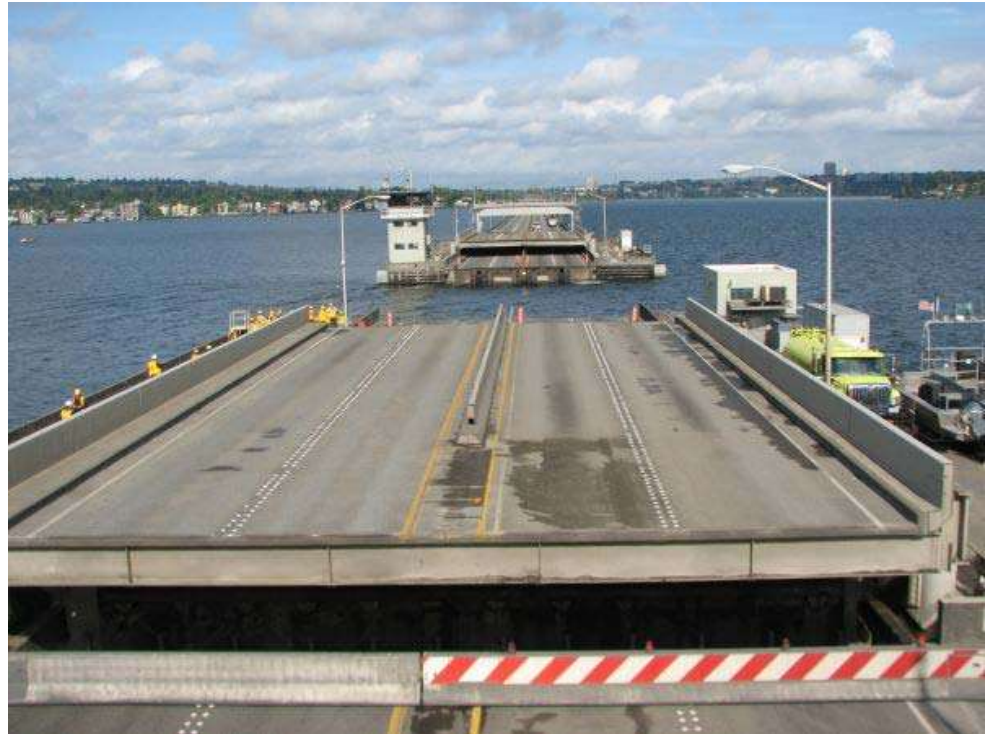
Figure 16.3.2 Movable Bridge Section of Evergreen Point Bridge, Seattle, WA
