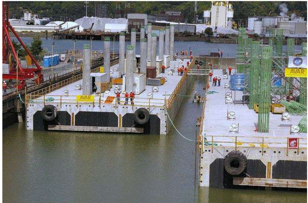
Figure 16.3.6 Concrete Pontoons Transported for Hood Canal Project
