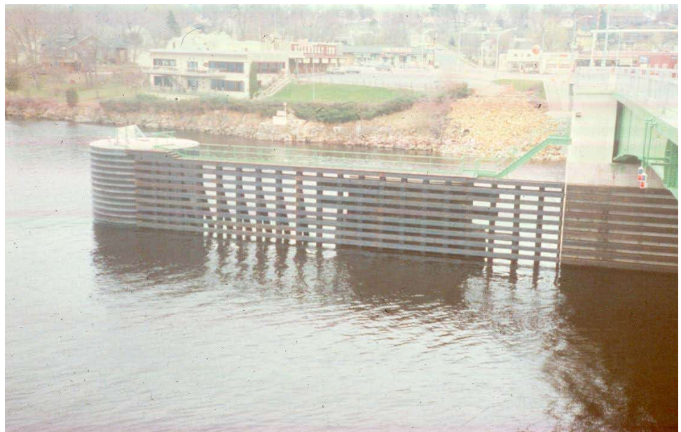
Figure 16.2.60 Pier Protection Systems – Dolphins and Fenders
