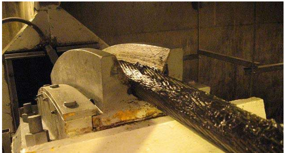
Figure 16.3.11 Anchor Cable Saddle
