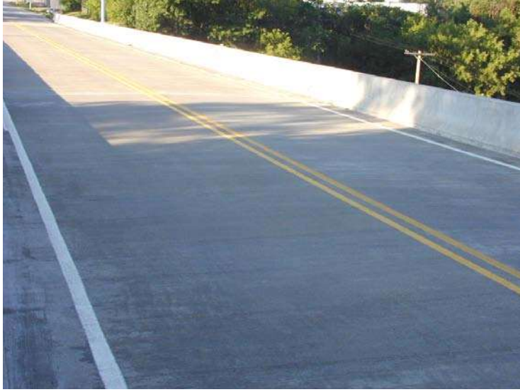
Photo No. 11 General Deck View
