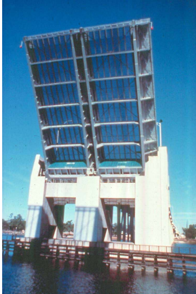
Figure 16.2.49 Transverse Locks on Underside can be Disengaged
