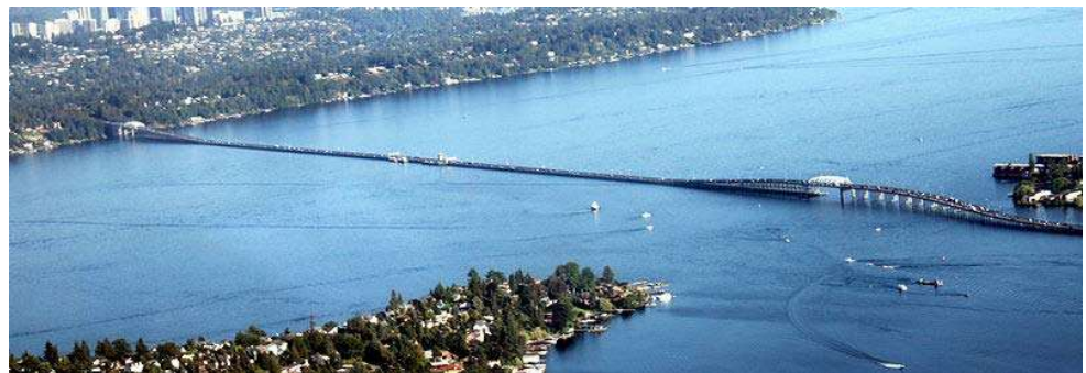
Figure 16.3.3 Elevated Section of Evergreen Point Bridge, Seattle, WA
