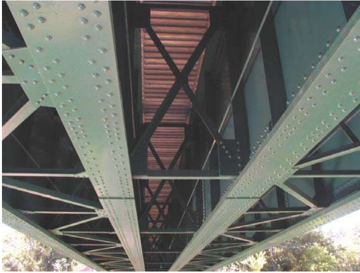
Photo No.9 General Underside View – Span 2
