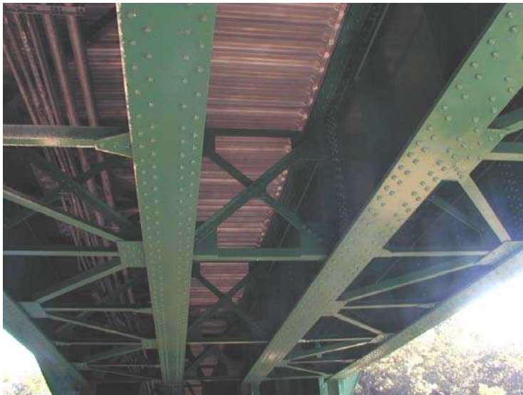
Photo No.8 General Underside View – Span 1
