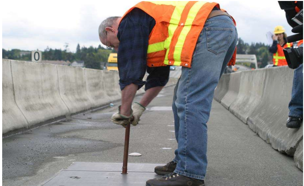
Figure 16.3.16 Inspector Opening Pontoon Access Hatch
